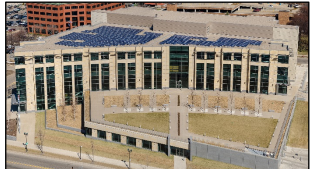
MINNESOTA SENATE BUILDING SOLAR PV INSTALLATION
